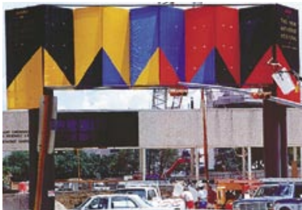
Methodist Hospital, Houston, TX Jobsite Entrance Arch, Applied Nylon on Steel Frame
